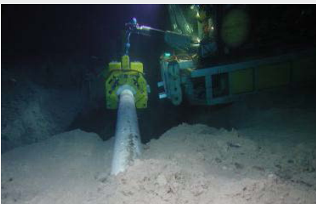
ROV-iT AT 500M DEPTH CONDUCTING TOFD & CORROSION MAPPING:
