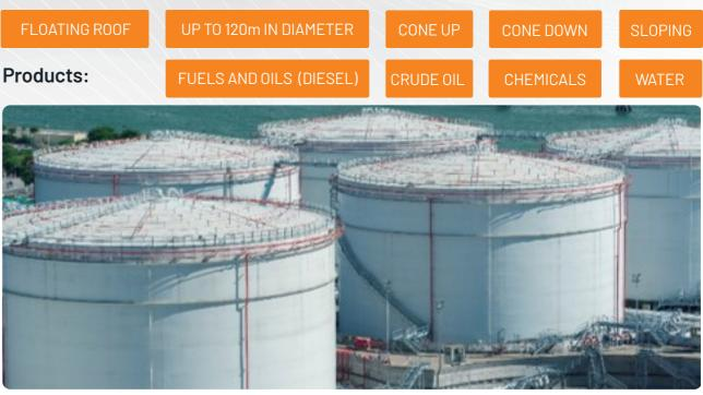
There can be potential application barriers when carrying out inspections if tanks have multiple internal obstructions on or near the floor, if tanks have internal floating roofs and fixed upper roof and/or if tanks have excessive sludge or have certain chemical content.
