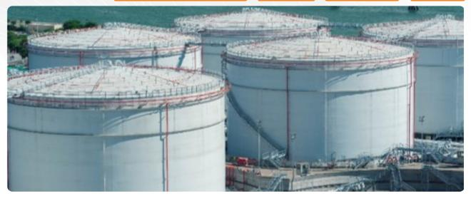
There can be potential application barriers when carrying out inspections if tanks have multiple internal obstructions on or near the floor, if tanks have internal floating roofs and fixed upper roof and/or if tanks have excessive sludge or have certain chemical content.
