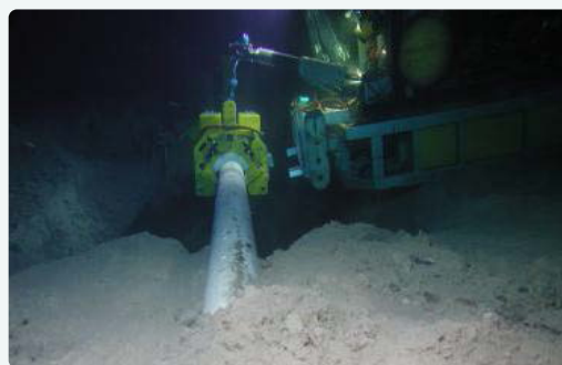
ROV-iT AT 500M DEPTH CONDUCTING TOFD AND CORROSION MAPPING:
