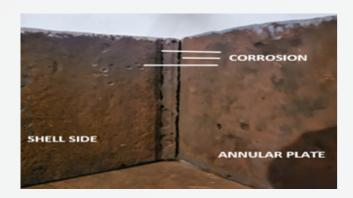
In addition to the A-ring application, an inspection from the shell side can be carried out, with the use of the fillet application, to get a full coverage of the fillet weld, especially the upper toe and HAZ for corrosion and/or cracking in that area.
