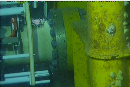
INSPECTION OF FLANGE WELD:
