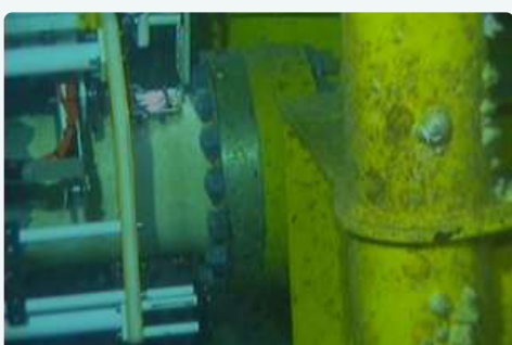
INSPECTION OF FLANGE WELD:
