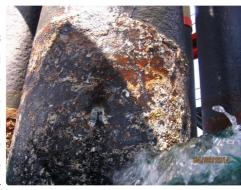
of marine growth and scale around the splashzone region. The conductor thickness was 22 mm for the first 2-3 sections and then increases up to 28 mm in the last section..
