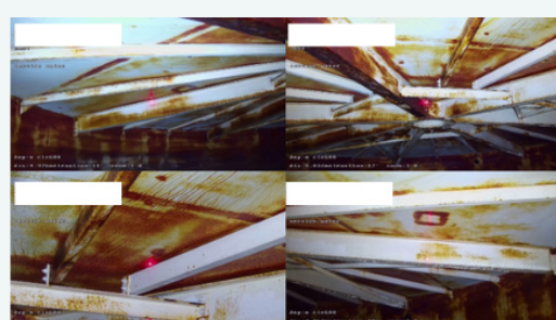
TANK ROOF PLATES & BEAMS
