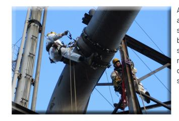
Any areas of degradation between the probes will affect the amplitude and arrival times of the received signals. Areas where evidence of degradation has been recorded can be ranked according to the severity of the signal disruption. This is a screening method allowing the condition of locations to be determined rapidly. The system has been used onsite in the UK, USA, Australia, and South Africa.
