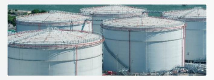
There can be potential application barriers when carrying out inspections if tanks have multiple internal obstructions on or near the floor, if tanks have internal floating roofs and fixed upper roof and/or if tanks have excessive sludge or have certain chemical content.
